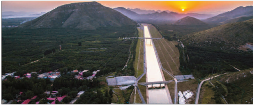
The Shunging section of China's South-North Water Diversion Project. Photo: china.org.cn
