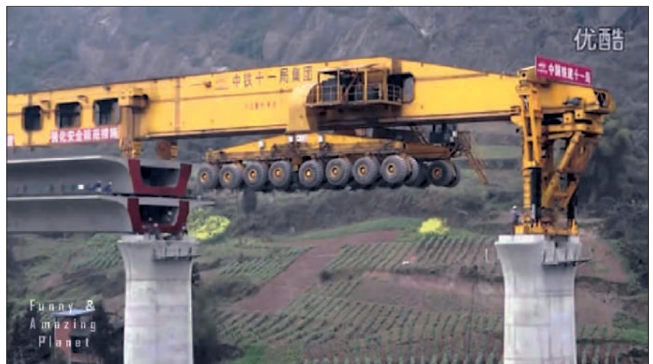
Machine in China enabling rapid placement of elevated trestles.
